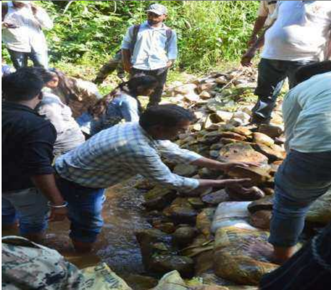
Dr G.B.Kale students and forest staff - Bandh Construction at Nakshatra Ban ,The Dnyanganga Wildlife Sanctuary
