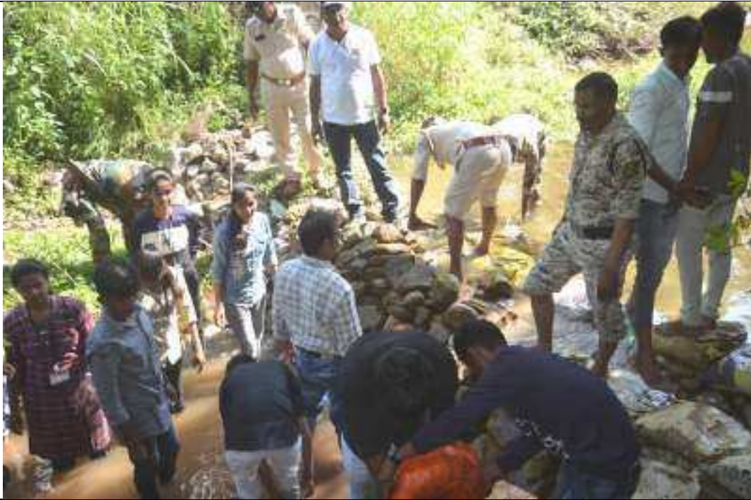
Dr G.B.Kale students and forest staff - Bandh Construction at Nakshatra Ban ,The Dnyanganga Wildlife Sanctuary
