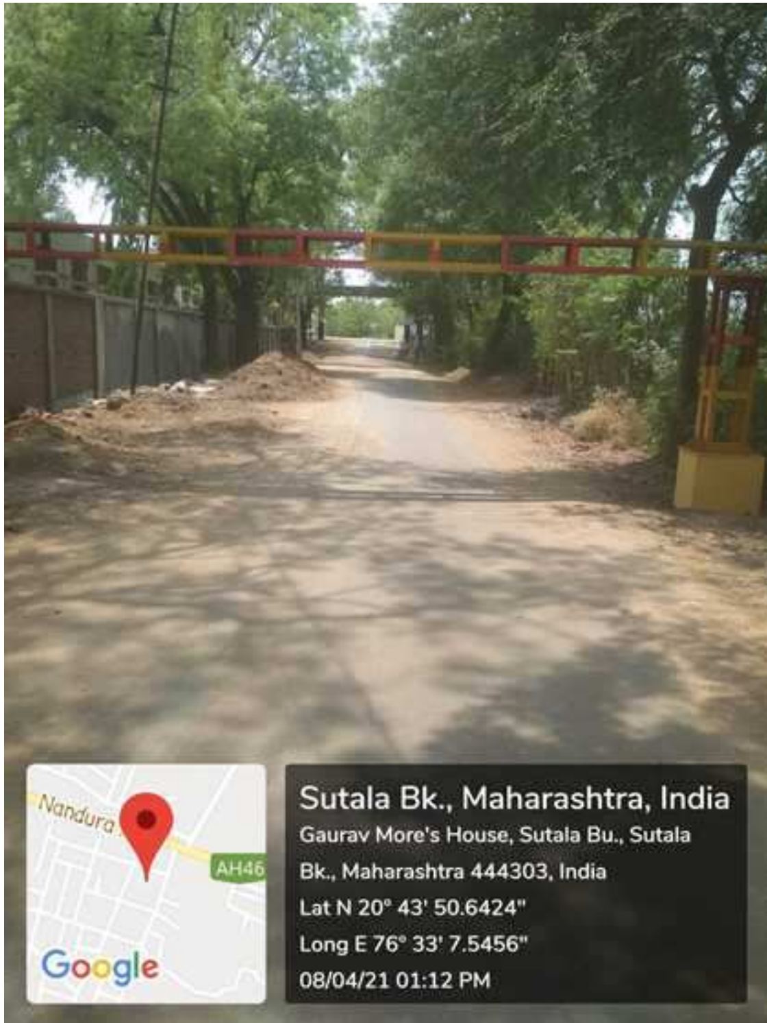
Barrier for restricted entry to heavy vehicles
